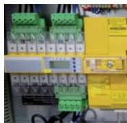
Transfer switching device ATICS®
